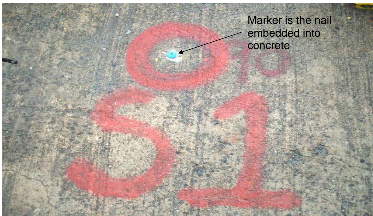
Station Marker is Nail on the Ground
